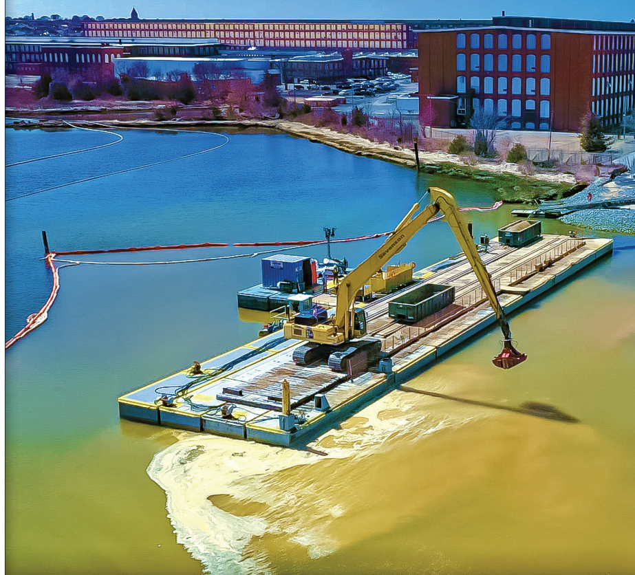
"Multi-layer cap placement near source area using a Komatsu PC450"
