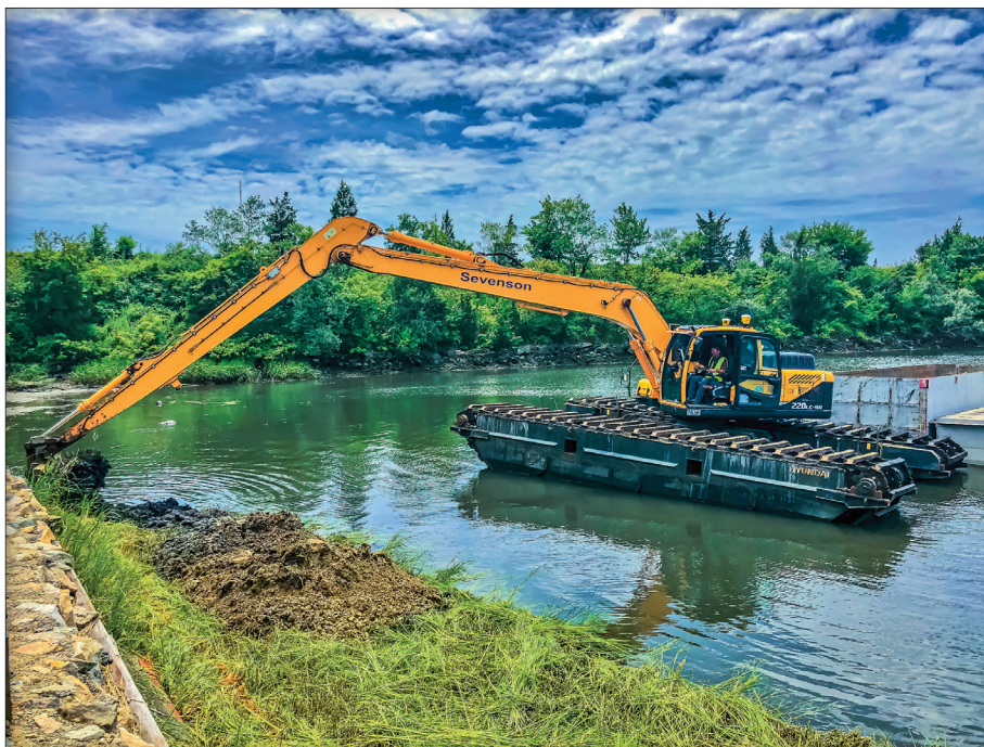
“Contaminated sediment removal in marsh area using a Hyundai 220LC Swamp Hoe”
