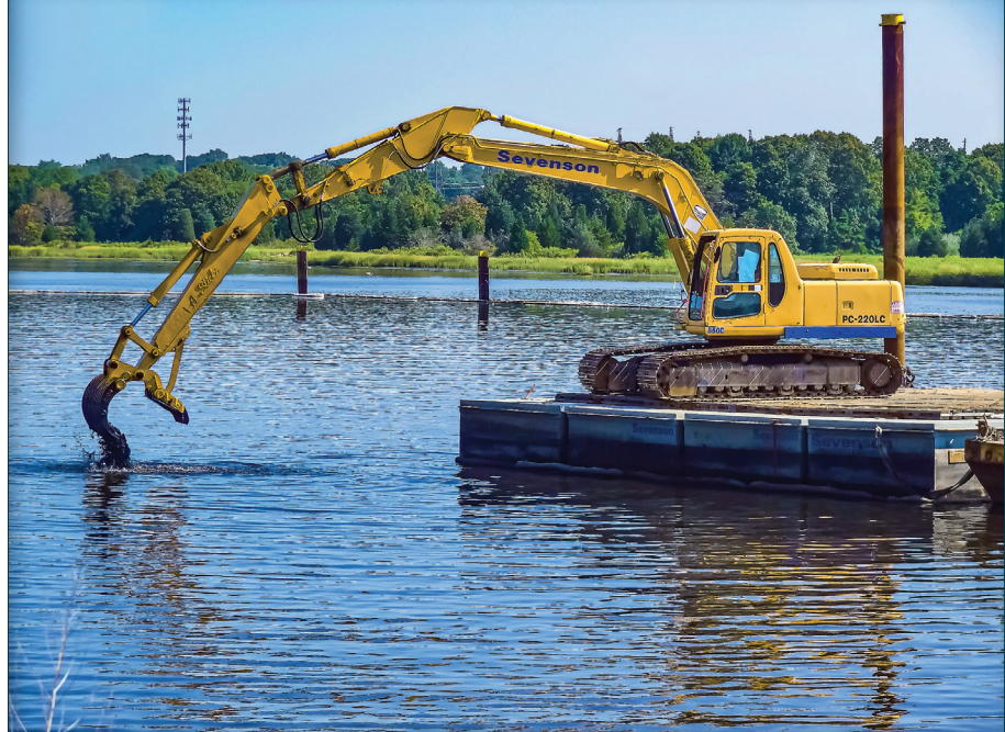
“Raking debris prior to hydraulic dredging”
