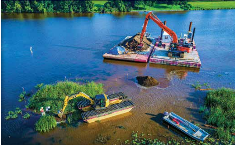
Floodplain backfill placement operations CLEAN UP
